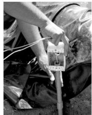
*Outdoor junction box for the pump-to-module connection.*
