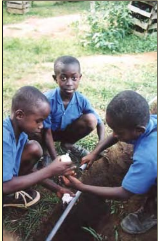
The kids at the school help glue PVC pipe. After just a few minutes of instruction, they were gluing like pros!
