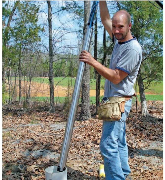
Installation of a Grundfos SQFlex submersible pump.
