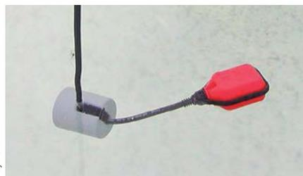
**A float switch hangs on a weight inside a storage tank.**
