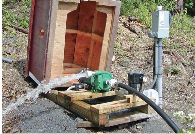
**A surface pump can move large amounts of water, but because it has a limited draw depth, it is not usually used in drilled wells.**
