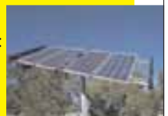
UTRK040 installation by Total Light & Power Pie Town, NM
