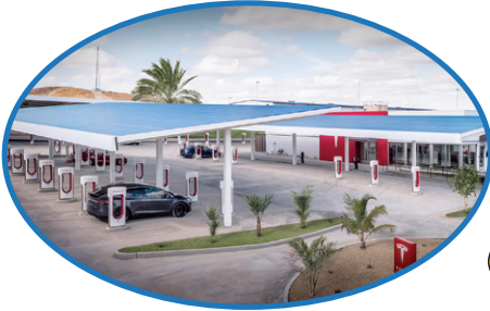
Tesla Charging Station
